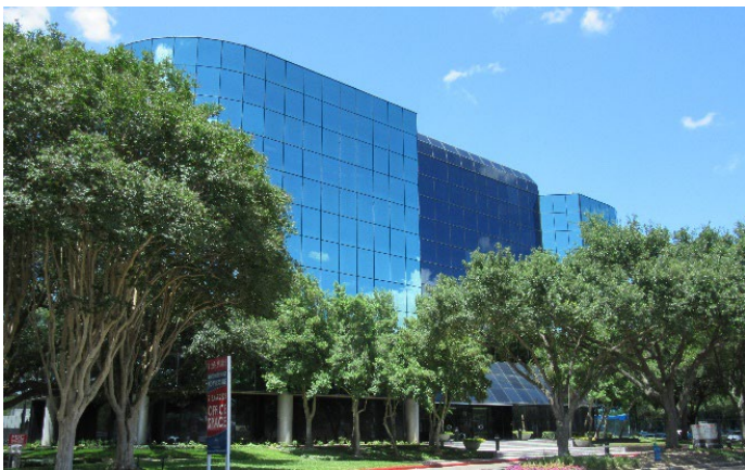
JBAH office is located on the 1 st floor of this 6-story building.
